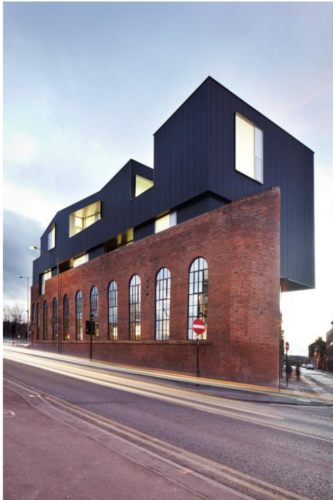
Shoreham street project/ PROJECT ORANGE
